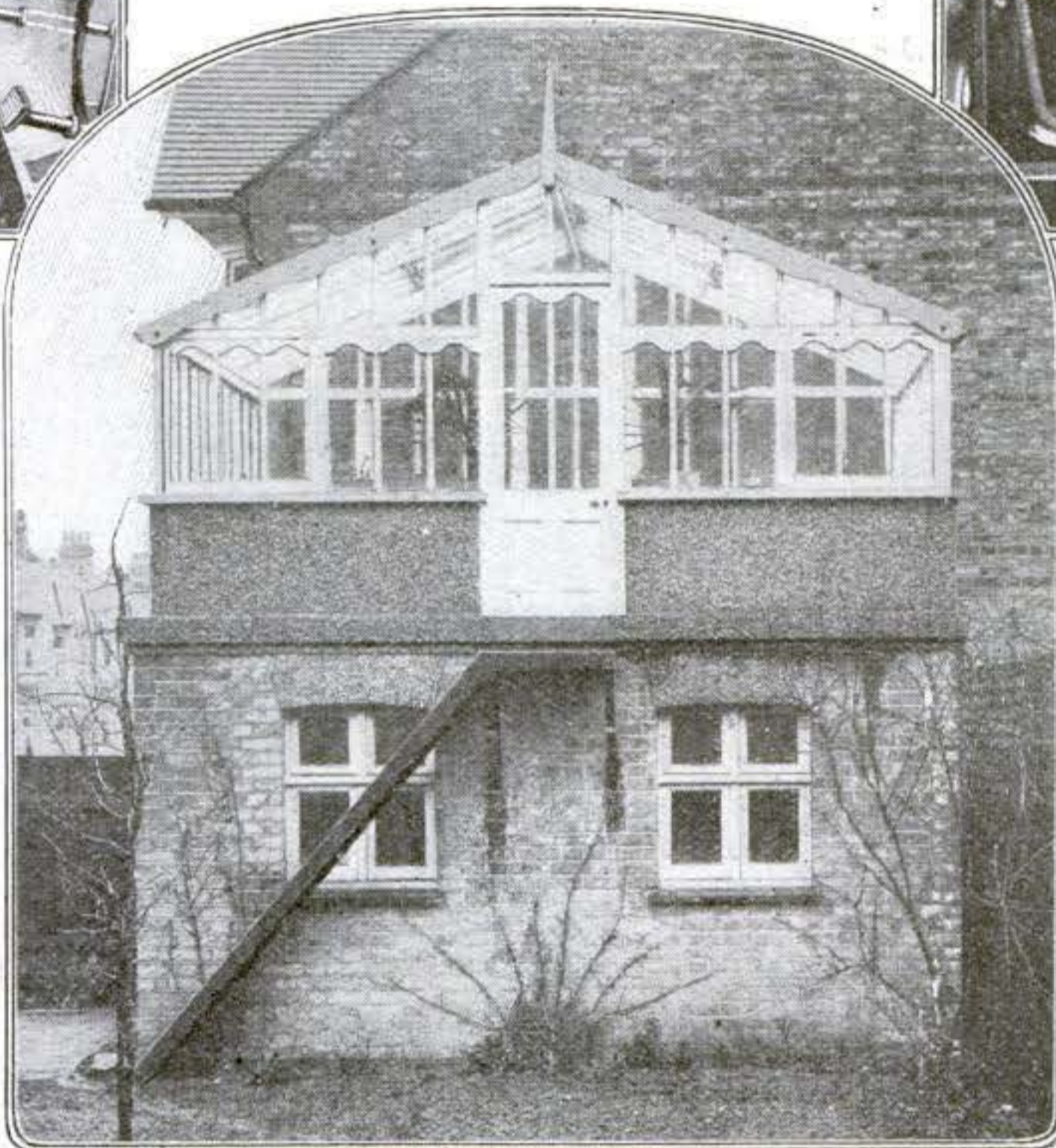
The combination of garage and conservatory is pleasing, and the double cost of tiles and roofing is eliminated
