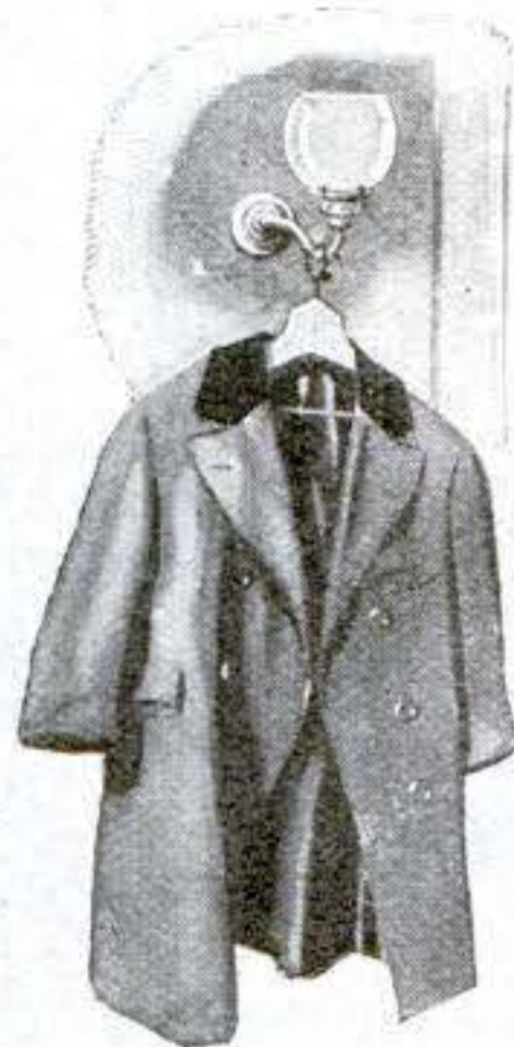
Many a leak has resulted from this unnatural use of the fixture
