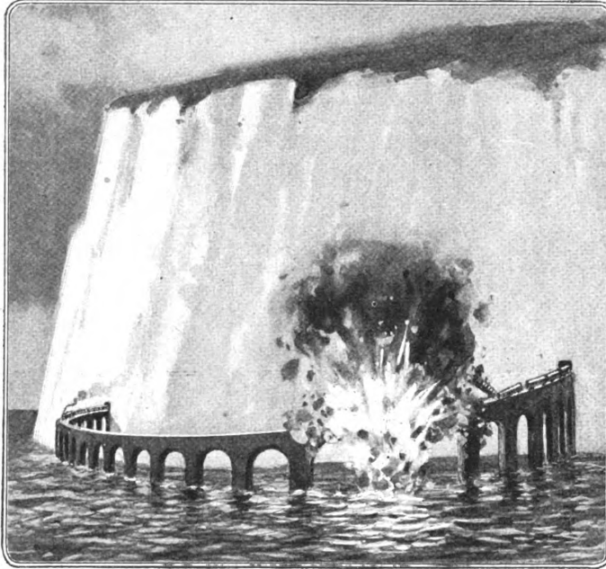
One of the early plans for the Channel tunnel provided an entrance at Dover in the form of a winding railway to climb to the top of the cliffs. What might have happened to this exposed entrance in time of war is suggested in the picture
